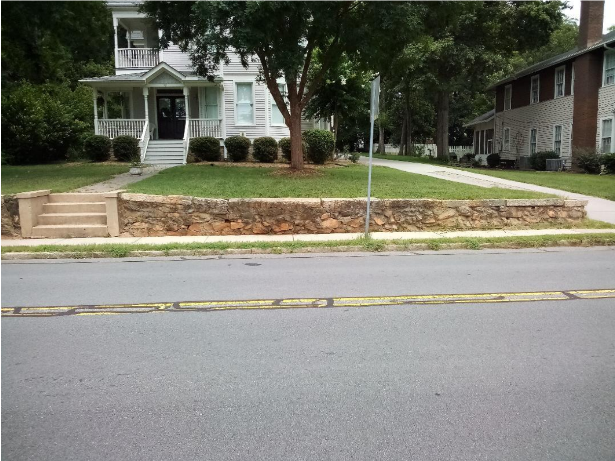
H-19-22 Existing Masonry Retaining Wall – Right Side
